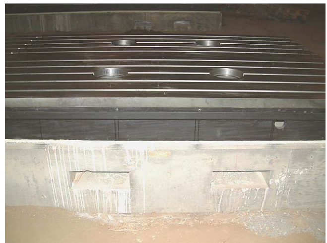
View on seismic mass with fluid trough bolted on below machined drip edge.
